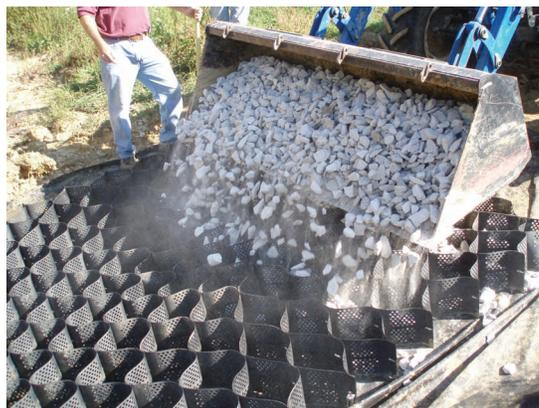
After preparing the site, geotextile fabric was laid down to act as a separation layer between the aggregate infill and the soft-bottomed streambed. With the fabric in place, the Geoweb system is stretched out, placed on top of the fabric and anchored into the streambed using rebar and clips which hook into the Geoweb. Limestone rock less than three inches is then used as the infill, as shown in the pictures to the left.
