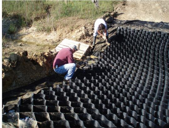
A new type of stream crossing using the Geoweb system was installed. The Geoweb system provides a stable stream crossing, allowing for livestock and farm equipment to cross safely. The Geoweb is a plastic, honeycomb-like surface designed to hold aggregate in place, even in flowing water. An engineered hole pattern in the system's cells helps to lock aggregate in the cells and resist aggregate washout.
