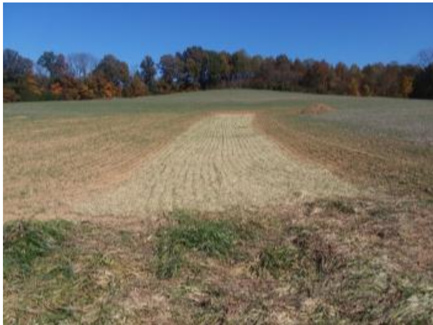
Straw blanket installed on grassed waterway extension. Energy from falling raindrops will be dispersed and erosion will be prevented.
