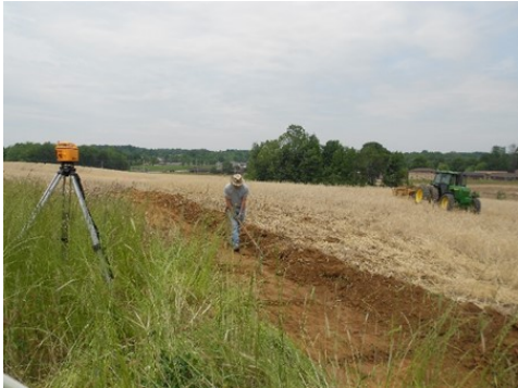
Field 7 diversion construction spring 2016
